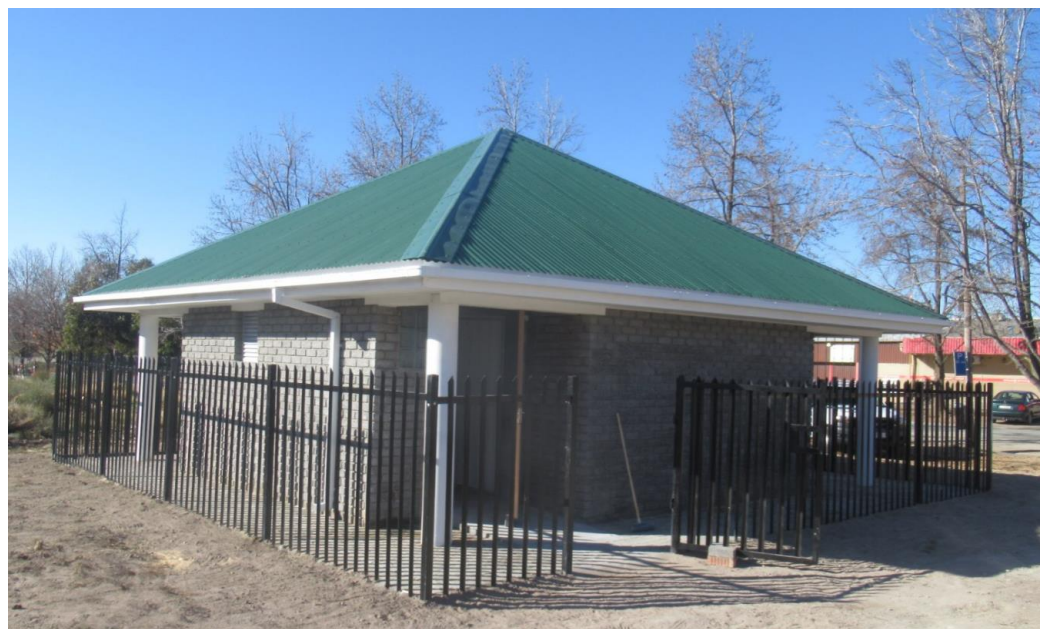
New public ablution facility at Op-Die-Berg
