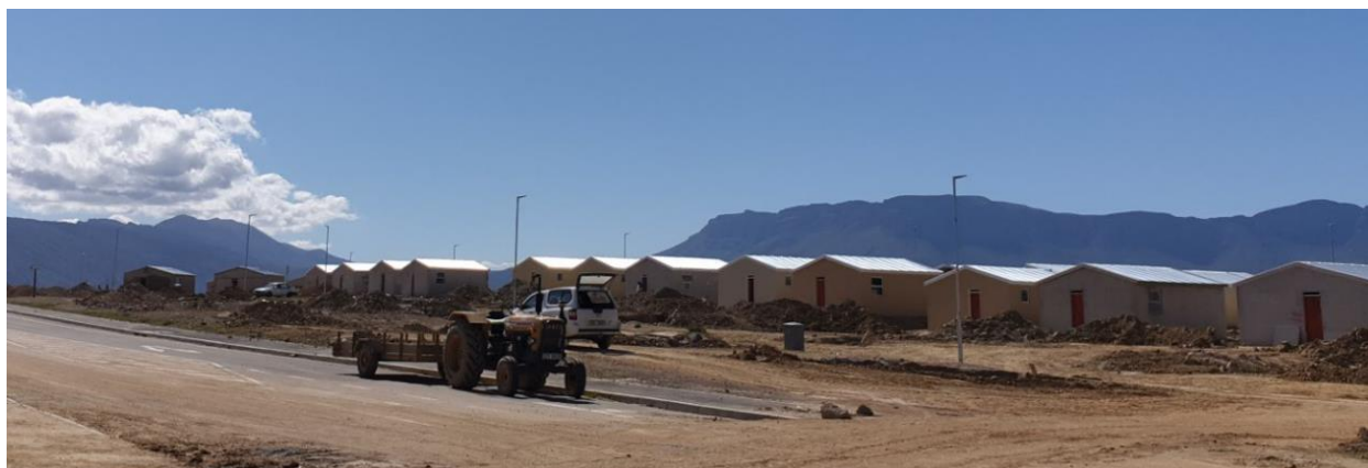
The 1 st phase of 229 houses was completed in Vredebes.
