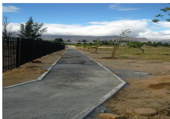
Bella Vista walkway
