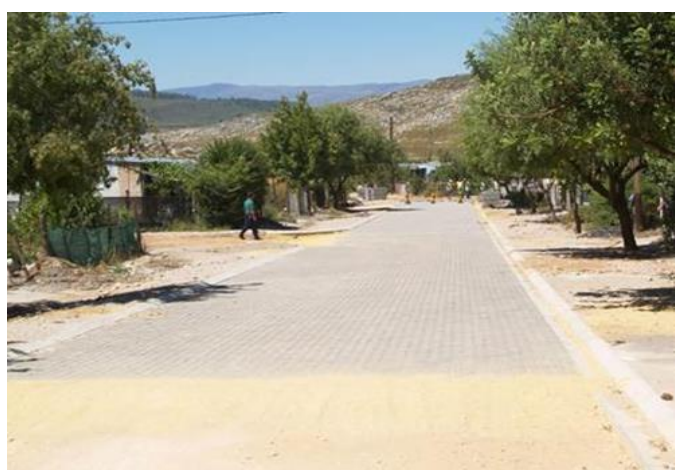
Op-die Berg road resurfacing
